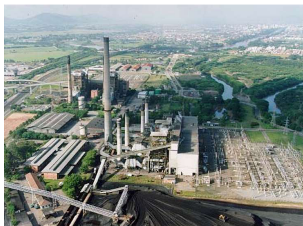
Figure 2: Jorge Lacerda Thermoelectric Complex, Capivari De Baixo -SC – Brazil.
